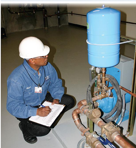
VISUAL AND AUDITORY INSPECTION
