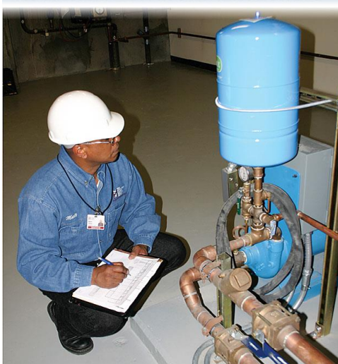
VISUAL AND AUDITORY INSPECTION
